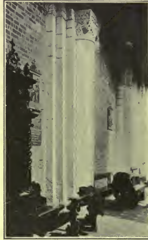
FIGURE 7.—EASTERNMOST ALTERNATE RESPOND IN NORTHERN SIDE AISLE.
