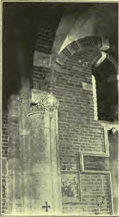
FIGURE 5. — EASTERNMOST RESPOND IN SOUTHERN SIDE AISLE; SHOWING CAPITAL AND SPRINGING OF THE VAULTS.
