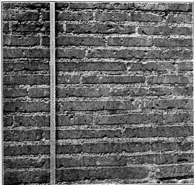
FIGURE 6. — ROOF-TILE FACING OF THE TIME OF HADRIAN. 2
