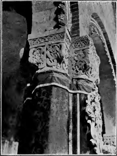
FIGURE 6.—CAPITAL OF THIRD PIER FROM WEST ON SOUTHERN SIDE OF NAVE.
