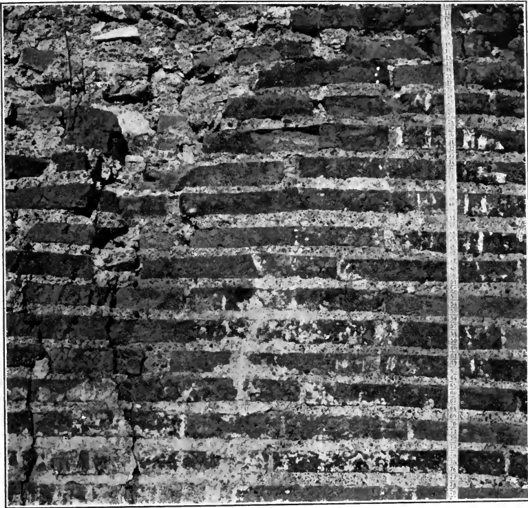
FIGURE 7.—BRICK FACING OF THE TIME OF SEPTIMIUS SEVERUS. 2
