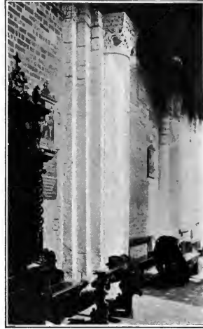
FIGURE 7.—EASTERNMOST ALTERNATE RESPOND IN NORTHERN SIDE AISLE.
