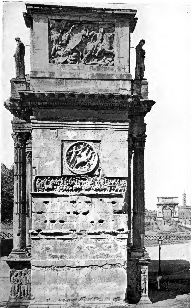
FIGURE 3.—EAST END OF THE ARCH OF CONSTANTINE. (With inserted medallion and frieze cut long after construction.)
