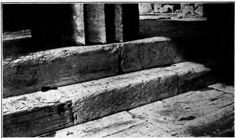
FIGURE 17. — RE-USED MARBLE BLOCKS. 1
