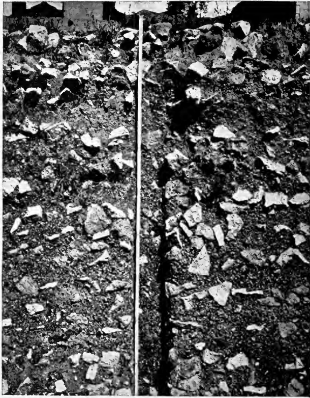
FIGURE 2.—AN UNFACED WALL OF OPUS CAEMENTICUM OF THE PERIOD OF NERO. 1
