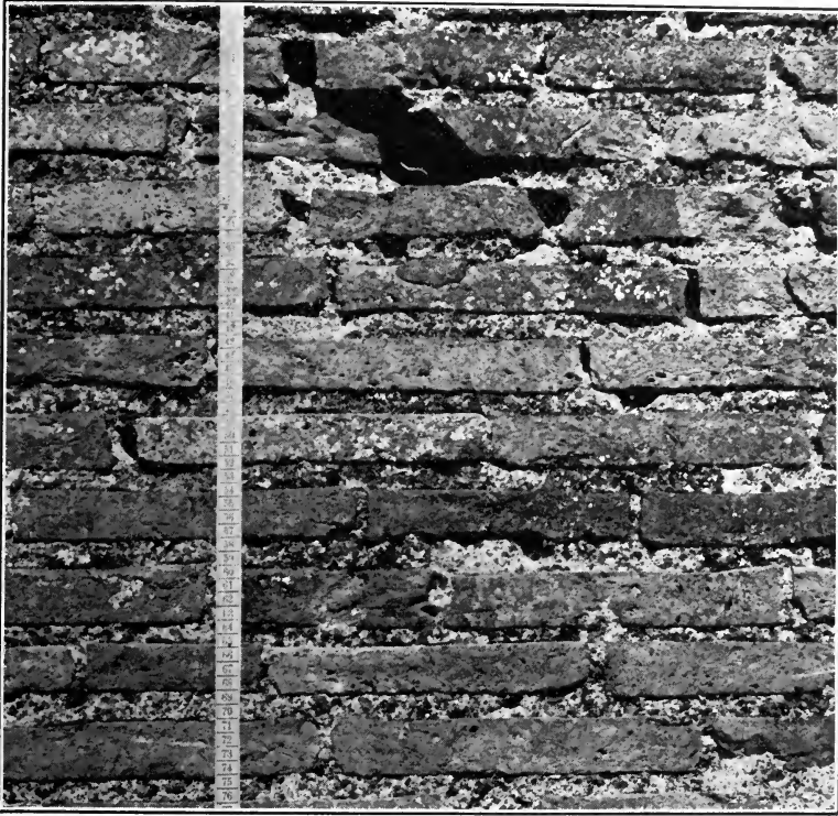
FIGURE 2. — FACING OF TRIANGULAR BRICKS OF THE TIME OF CLAUDIUS. 2
