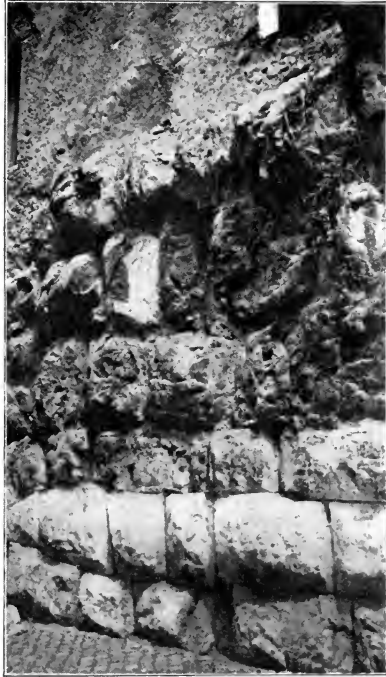
FIGURE 7.—PORTION OF INNER CIRCUIT OF WALL (Fig. 1, 24) IN VIA CORRADINI
