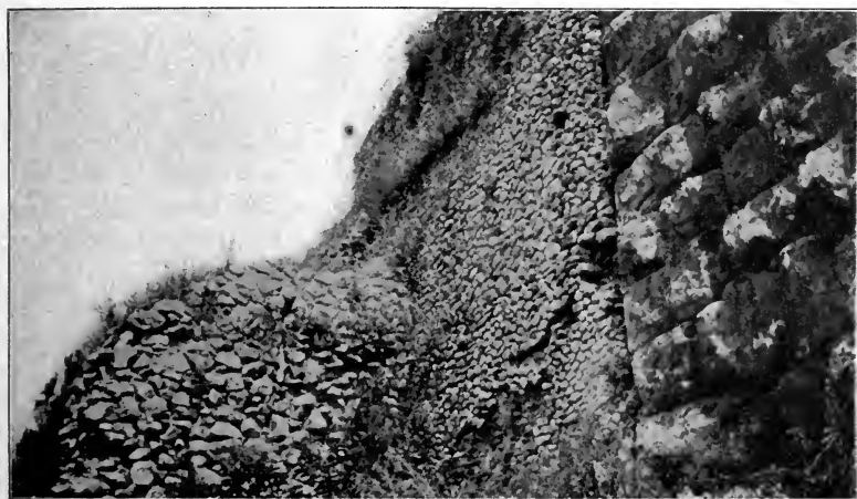
FIGURE 6.—NORTHWESTERN CORNER OF BASTION (FRAGMENT 14) SHOWING LATER ADDITION (a)
