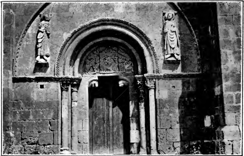
FIGURE 2.—LEON; S. ISIDRO; PORTAL OF SOUTH TRANSEPT
