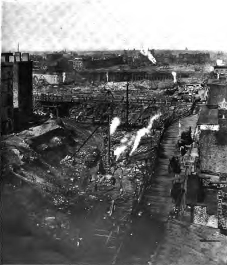
Excavating for the Pennsylvania Station
