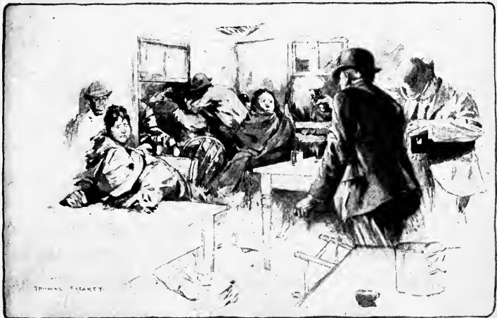
“The tenants bolted through the windows.”
