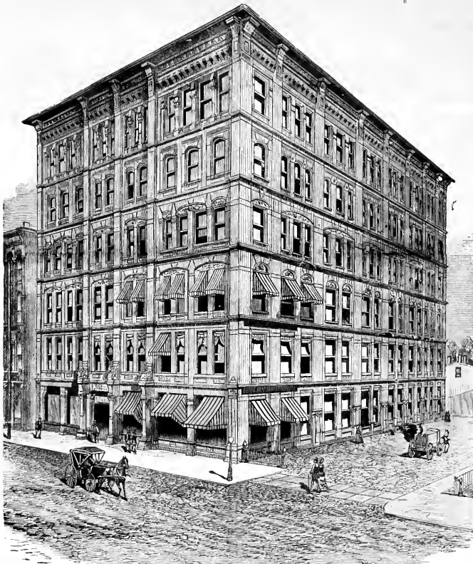
The Coal and Iron Exchange Building, Buffalo, N. Y., elevator accommodations, in which Clark's Business College is located.
