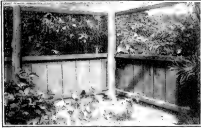
FIGURE 3-A.—Corner of New Jersey type stationary pen, showing employment of boards in constructing sides to prevent alarming of birds.
