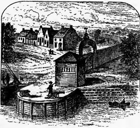
THE EAST RIVER GATE AND BLOCKHOUSES OF THE STOCKADE
