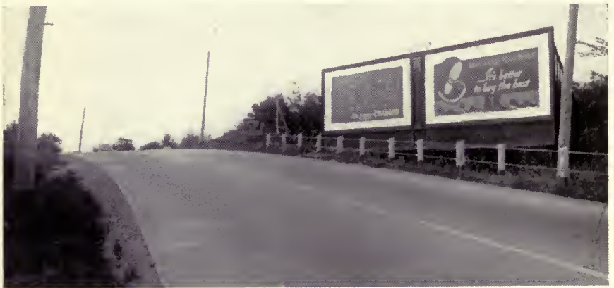
Billboards on an abrupt crest provide an unnecessary distraction to the driver Courtesy Roadside Bulletin
