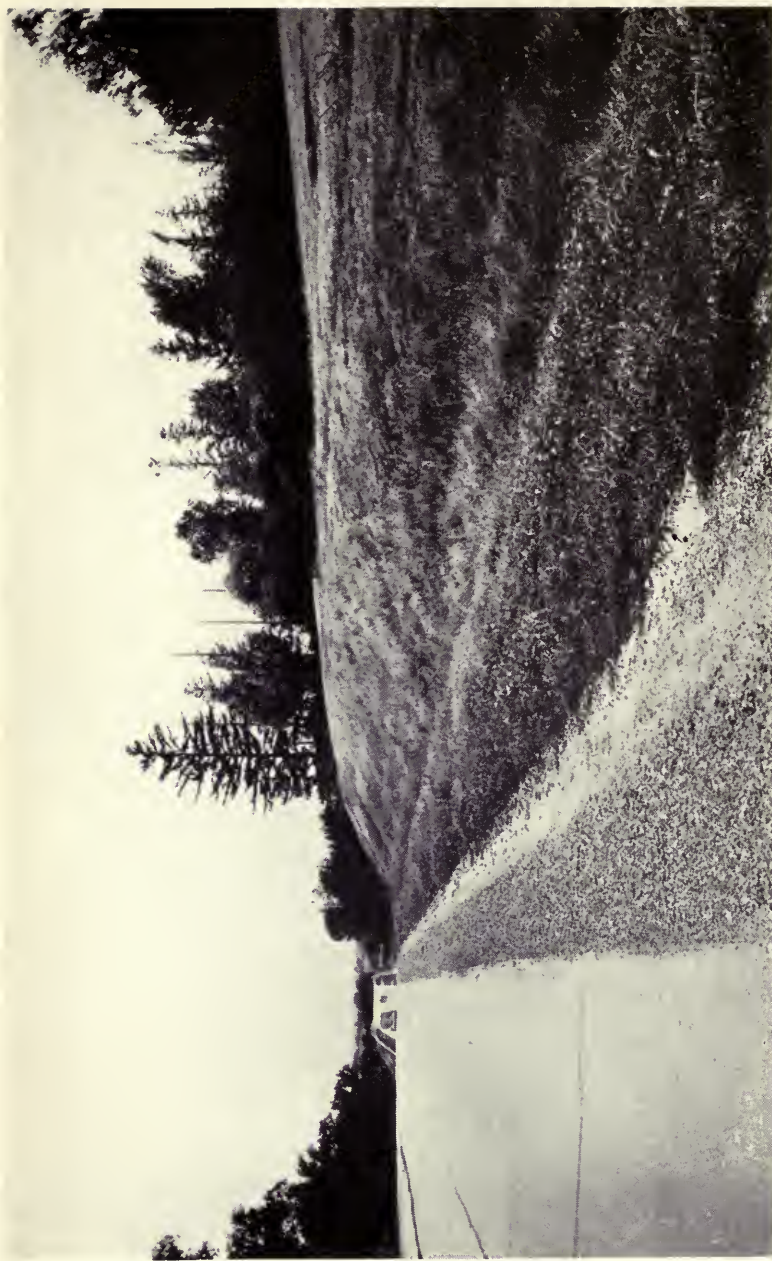
Natural sodding of the slopes merges Wisconsin's highways into the surroundings with beauty as well as lowered maintenance cost
