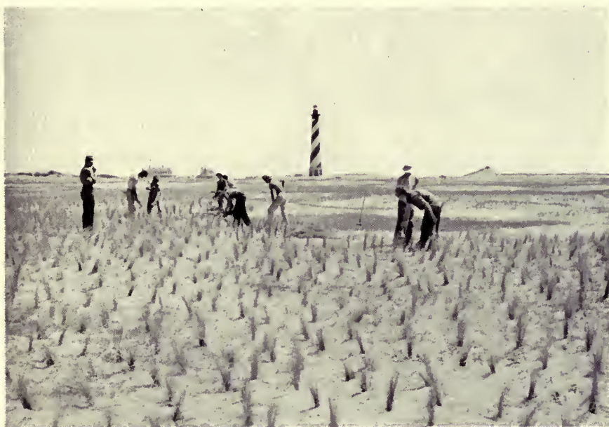
Grass planting to control wind erosion of Cape Hatteras Beach Courtesy U. S. Department of the Interior
