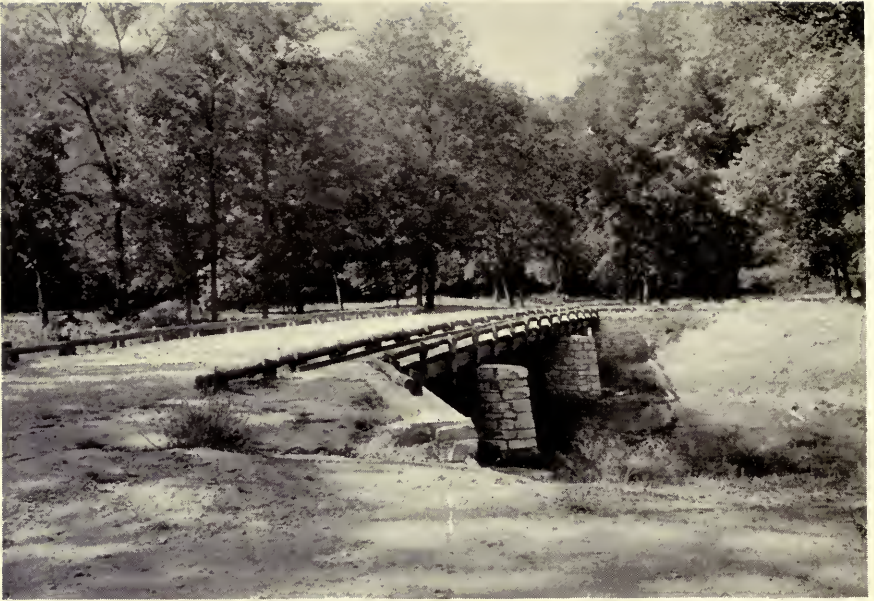
Combined truck and foot bridge in Backbone State Park, Iowa Courtesy U. S. Department of the Interior
