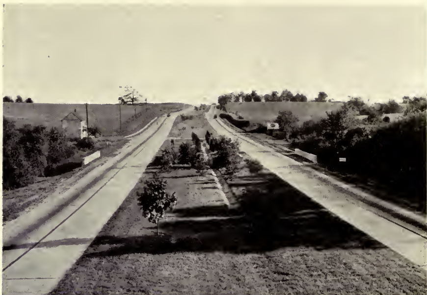
Divided roadway newly planted around a bridge in New Castle County, Delaware Photograph from Delaware State Highway Department
