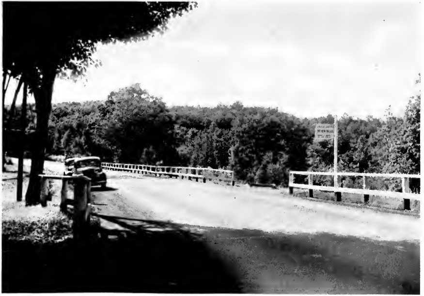
Entrance to a roadside park in Connecticut. Courtesy U. S. Bureau of Public Roads
