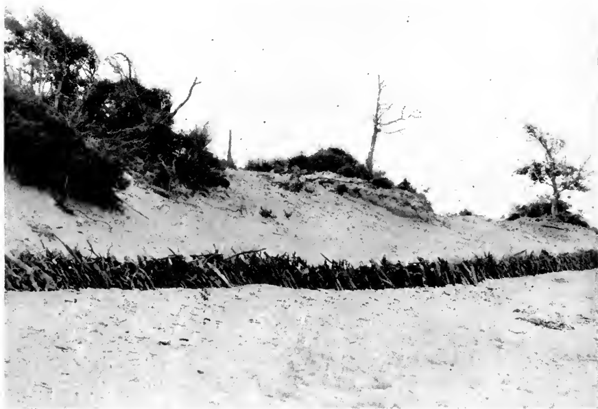
Sand fence constructed by WPA in beach erosion control Courtesy U. S. Department of the Interior
