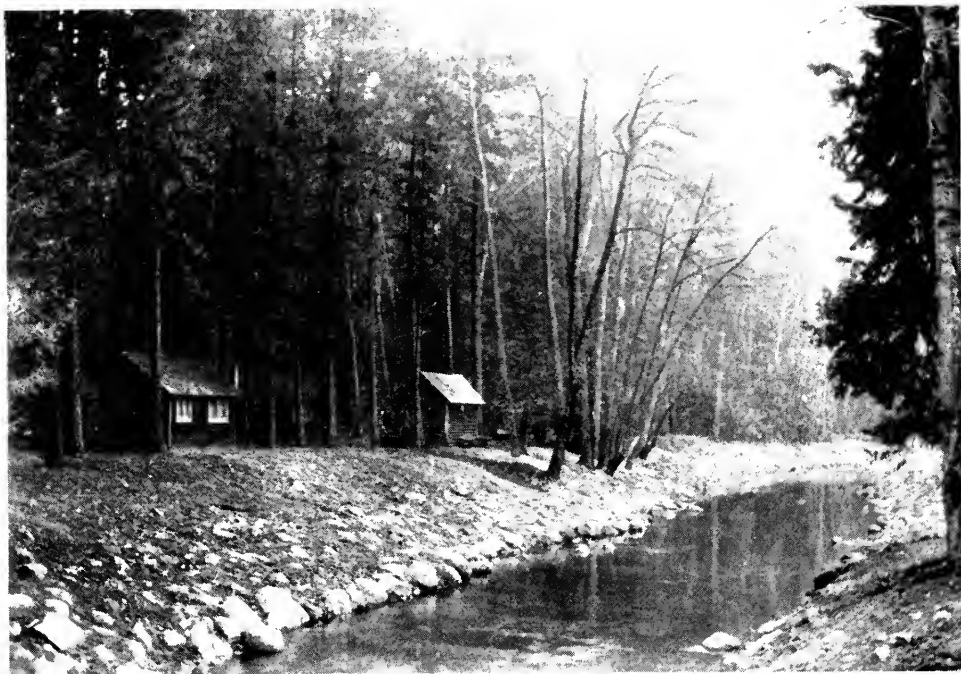
A flood-control project executed by the CCC in the state parks Photograph courtesy American Forests
