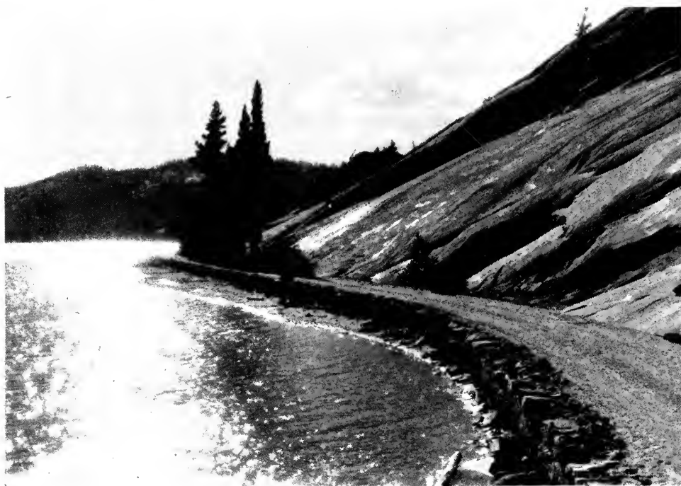
Wilderness beauty in the state parks made accessible by trails and roads constructed by the CCC Photograph courtesy American Forests
