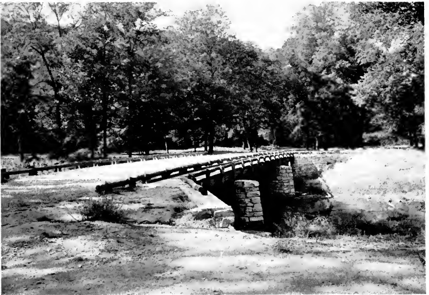
Combined truck and foot bridge in Backbone State Park, Iowa Courtesy U. S. Department of the Interior
