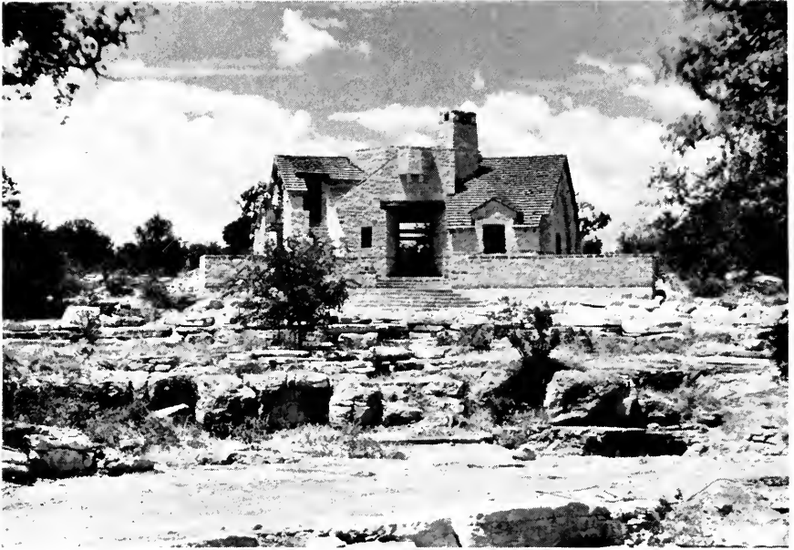
Refectory Building, Longhorn State Park, Texas Courtesy U. S. Department of the Interior
