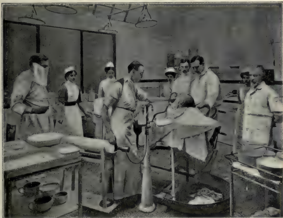
FIG. 91.—Arrangement, at the National Hospital, Queen Square, for Anaesthetization and Oxygenation of the Patient. The Vernon Harcourt regulator is fixed on the conical stand, the chloroform bottle being in a water-bath. The oxygen supply from the horizontal cylinder is readily regulated by the anaesthetist, Dr. Powell. Prof. Theodor Kocher of Berne, who happened to be visiting the hospital at the time, stands at the right of the photograph. (From Sir Victor Horsley's Address at the Toronto Meeting of the British Medical Association, 1906, on "The Technique of Operations on the Central Nervous System.")
