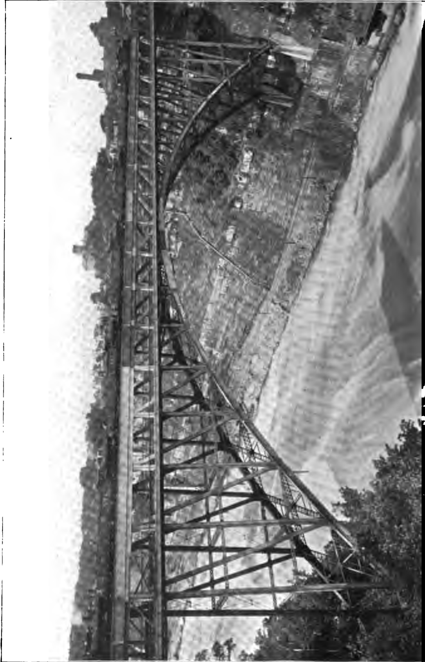
The above cut is a reproduction of a photograph taken on day of testing steel arch across Niagara River, completed by this Company in 1907. Fifteen locomotives and loaded freight cars, making an aggregate load of 2,500 tons. Clear span of arch, 540 feet. Total length, 1,080 feet. Upper floor, double track railway; lower floor 45 ft. highway and two sidewalks. LIGHT AND HEAVY STEEL ARCH in silhouette.
