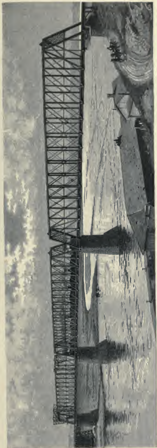
Truss Bridge of the Northern Pacific Railway over the Missouri River at Bismarck, Dak.—Testing the central span.
