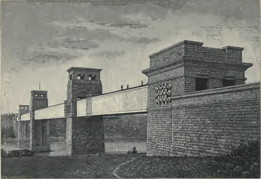
The Britannia Tubular Bridge over the Menai Straits, North Wales.
