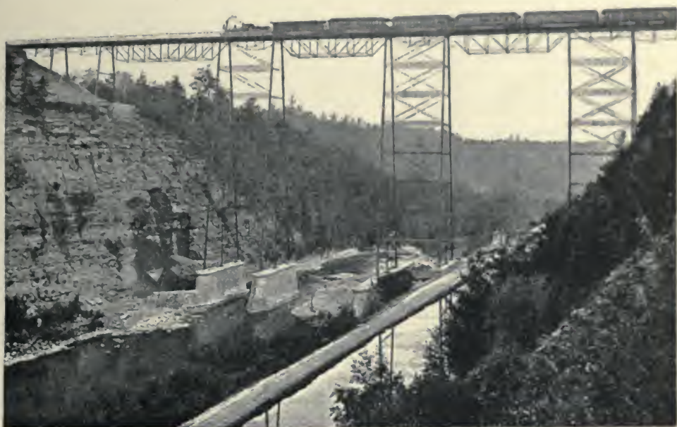
The New Portage Viaduct.
