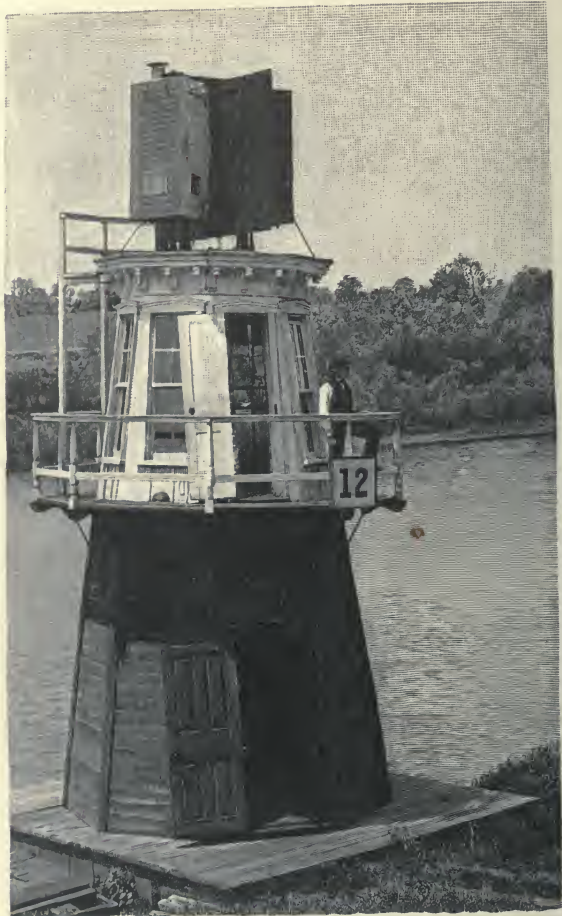
Old Signal Tower on the Philadelphia & Reading, at Phoenixville.
