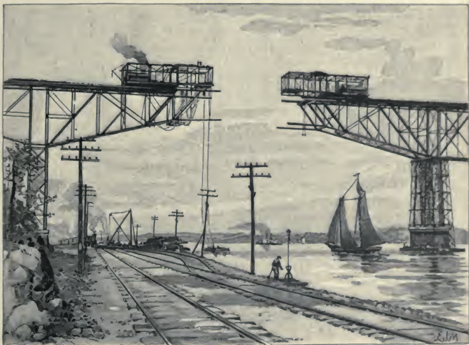
Erection of a Cantilever.
