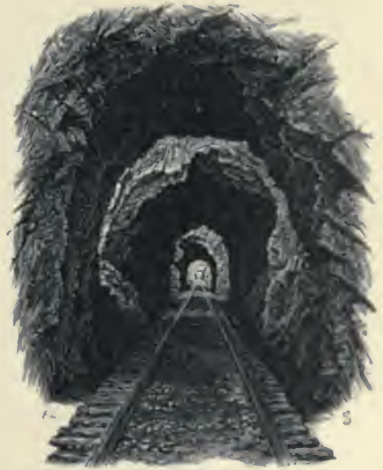
A Series of Tunnels.
