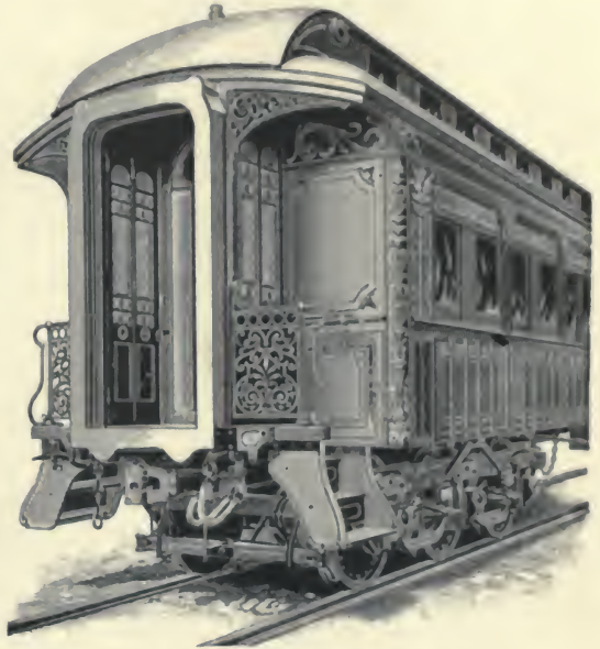
End View of a Vestibuled Car.
