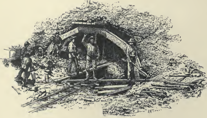
Beginning a Tunnel.
