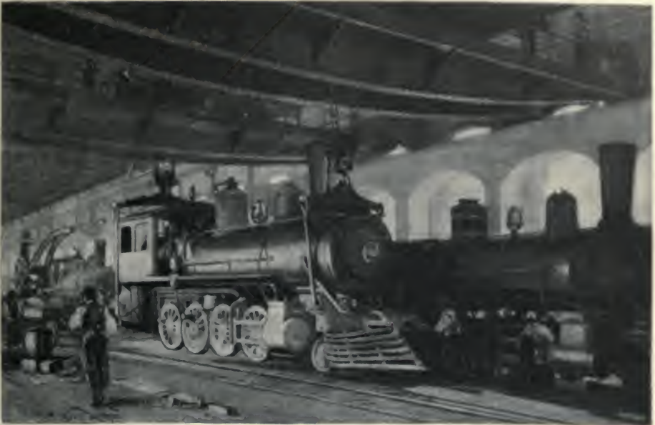
Fig. 38.—Interior of Erecting Shop, Showing Locomotive Lifted by Travelling Crane.
