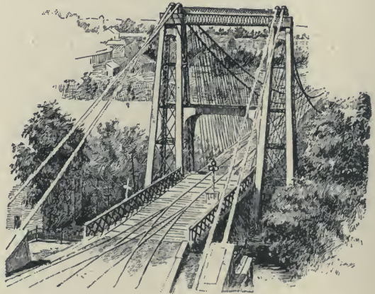
The New Iron Towers of the Same.
