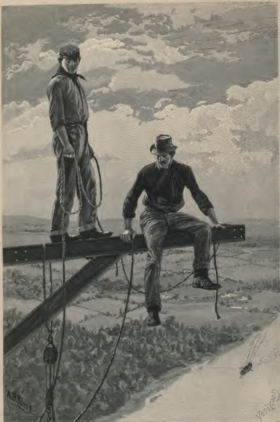
THE LAST SPAN—READY TO JOIN.
