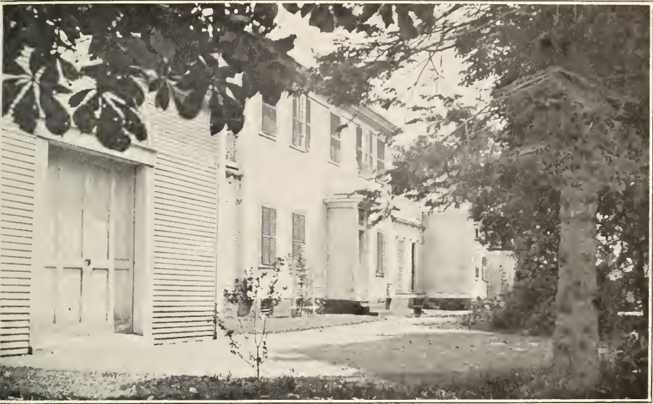
WEST APPROACH AND ENTRANCE DE WOLF-MIDDLETOWN HOUSE, BRISTOL, R. I. BUILT IN 1808.
