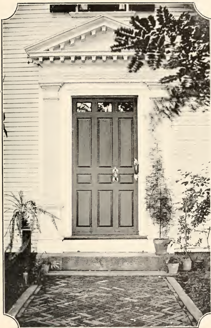
DOORWAY, MEANS' HOUSE, AMHERST, N. H.
