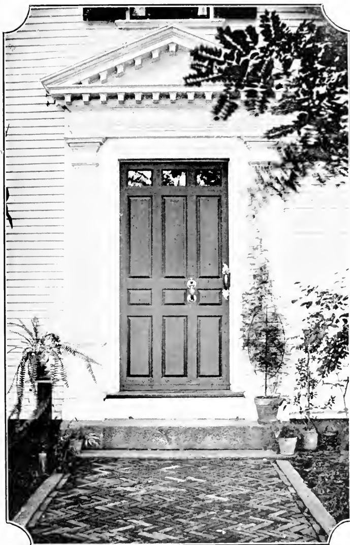
DOORWAY, MEANS' HOUSE, AMHERST, N. H.
