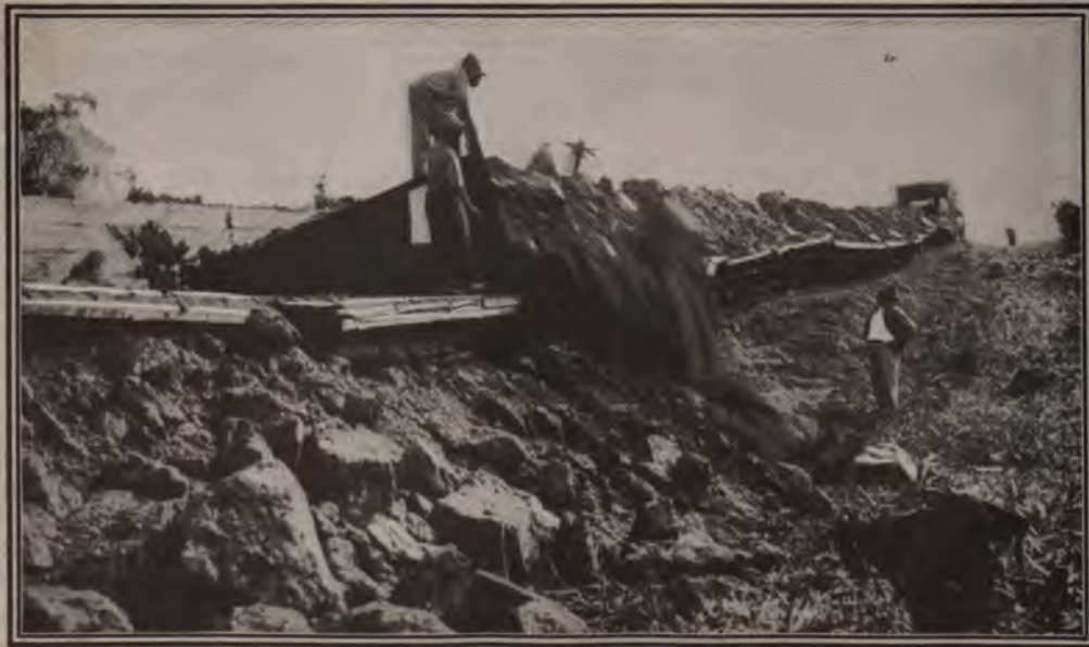
UNLOADING A DIRT TRAIN AT THE TABERNILLA DUMPS.
