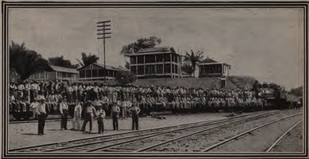
A TYPICAL WORK TRAIN.
