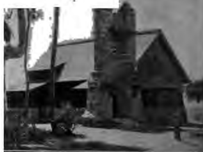
Santa Monica Hotel, Santa Monica, Cal. A. R. Benton, Architect, Los Angeles. Stained with Cabot's Shingle Stains.
