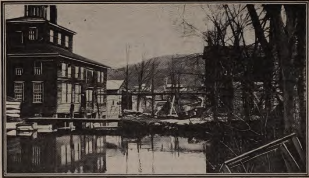
ONE OF MANY ABANDONED MILL-DAMS THAT MIGHT BE UTILIZED IN PRODUCING ELECTRIC CURRENT.
