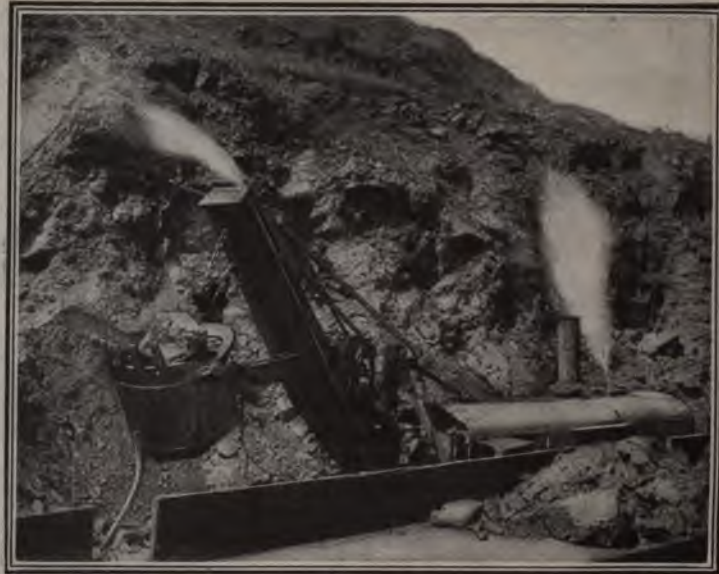
A STEAM SHOVEL AT WORK IN CULEBRA CUT.
