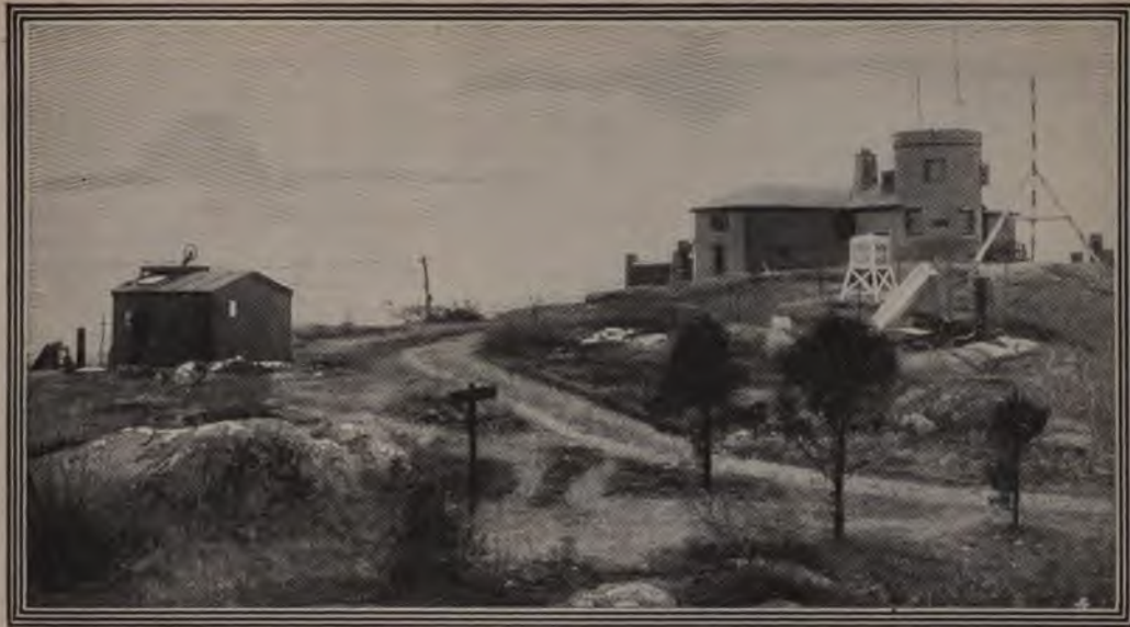
THE BLUE HILL METEOROLOGICAL OBSERVATORY, MILTON, MASS. (The building on the left contains power plant and windlass for winding in the kites.)
