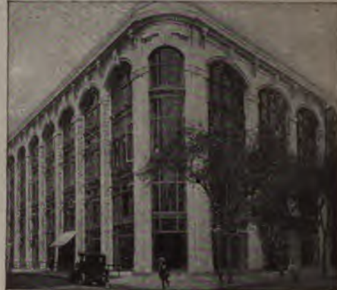
Packard Garage Building, New York City, N. Y.
