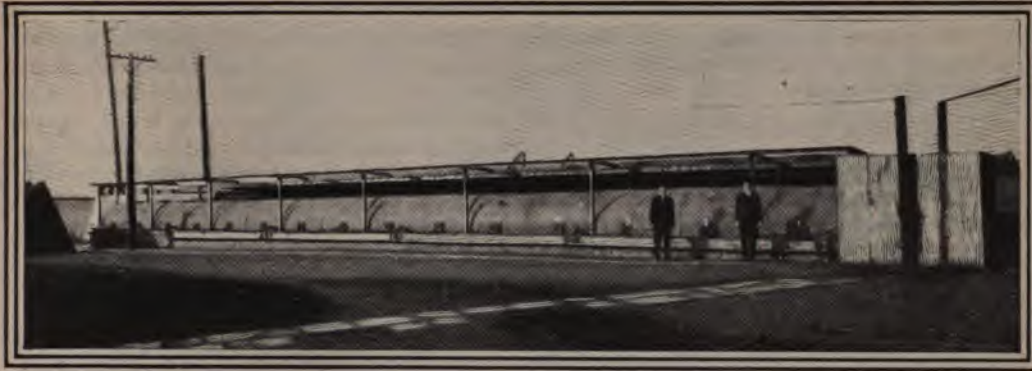
A SIDE VIEW OF THE EXPLOSIVES GALLERY AT PITTSBURG, SHOWING PORT-HOLES AT SIDE.
