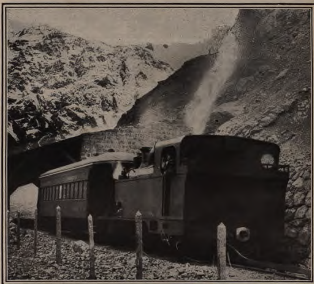
AN AVALANCHE SHED ON THE TRANSANDINE LINE.
