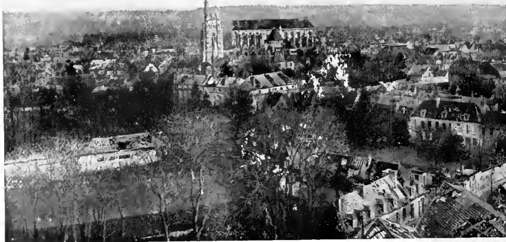
SOISSONS IN NOVEMBER, 1918. NOTE THE SEPARATION OF THE CATHEDRAL TOWER FROM THE NAVE.
