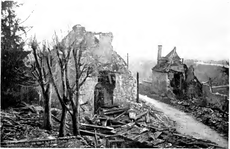
RUINED CHURCH AT MONT-ST.-PÈRE.
