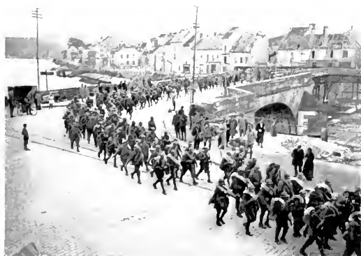
ITALIAN INFANTRY CROSSING CHÂTEAU-THIERRY BRIDGE, OF WHICH ONLY ONE ARCH REMAINS.
