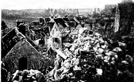
OULCHY-LE-CHÂTEAU SEEN FROM THE TERRACE.
