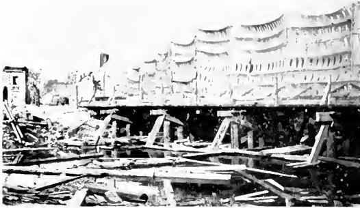
TEMPORARY BRIDGE OVER THE VESLE. "CAMOUFLAGED" DURING THE OPERATIONS.
