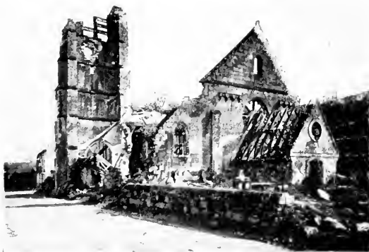
RUINED CHURCH OF ST. BANDRY.
