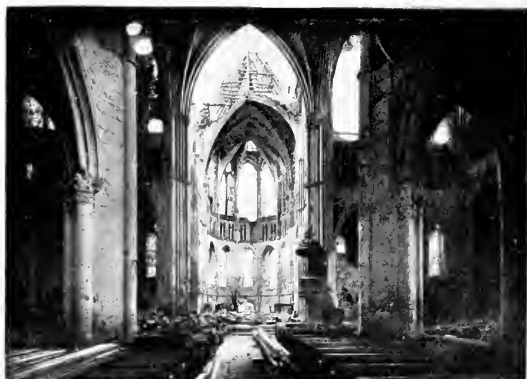
THE NAVE AND CHOIR OF ESSOMMES CHURCH, WHOSE VAULTING HAS FALLEN IN.
