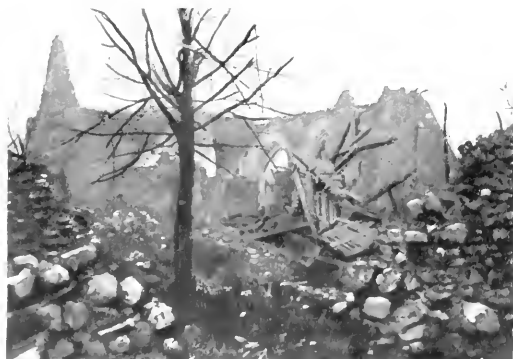
DOMMIERS CHURCH IN RUINS.
