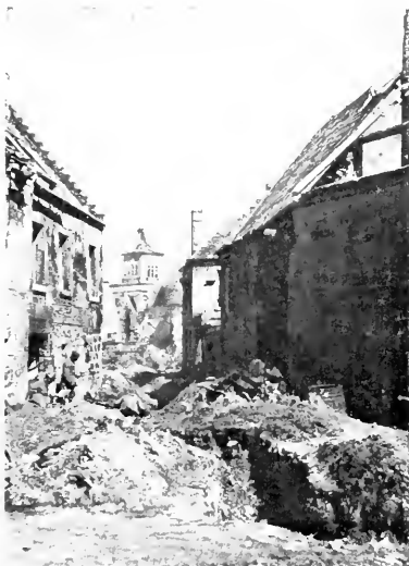
COMMUNICATING TRENCH IN ONE OF THE STREETS OF CROUY IN 1916.
