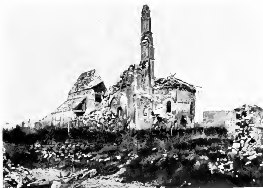
RUINED CHURCH OF OULCHY-LA-VILLE.
