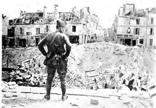
CHÂTEAU-THIERRY BRIDGE AFTER IT WAS BLOWN UP.
