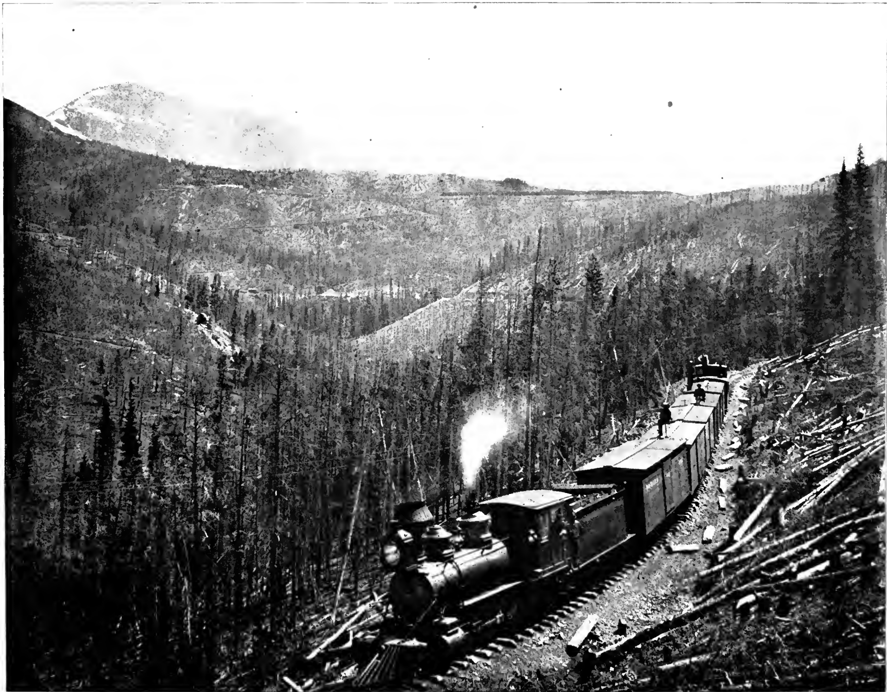
WEST SIDE OF MARSHALL PASS, SHOWING THE WINDING DESCENT OF THE ROAD.
