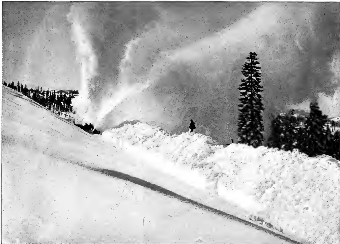
A ROTARY SNOW-PLOW CUTTING THROUGH A BLOCKADE ON THE SIERRAS.
