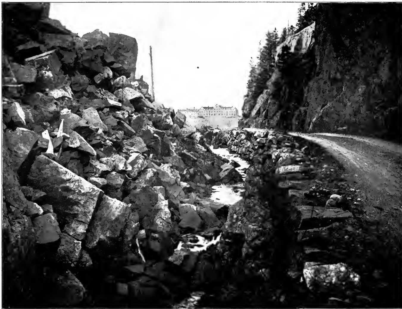
CRAWFORD HOUSE NOTCH, NEW HAMPSHIRE.
