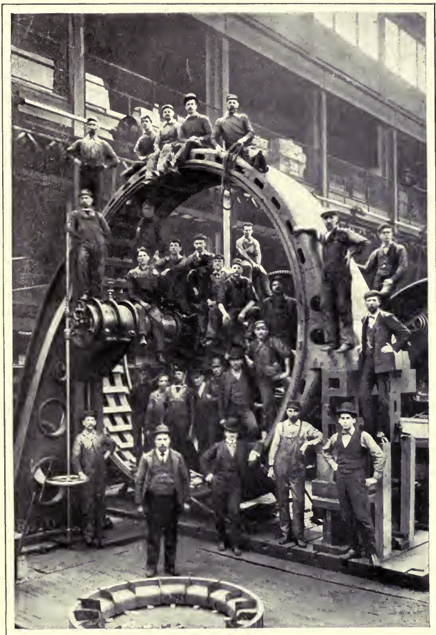
A HUGE GENERATOR FIELD AT THE WESTINGHOUSE WORKS
