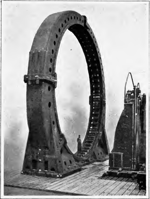
A COLOSSAL WESTINGHOUSE ROTARY FIELD GENERATOR.
