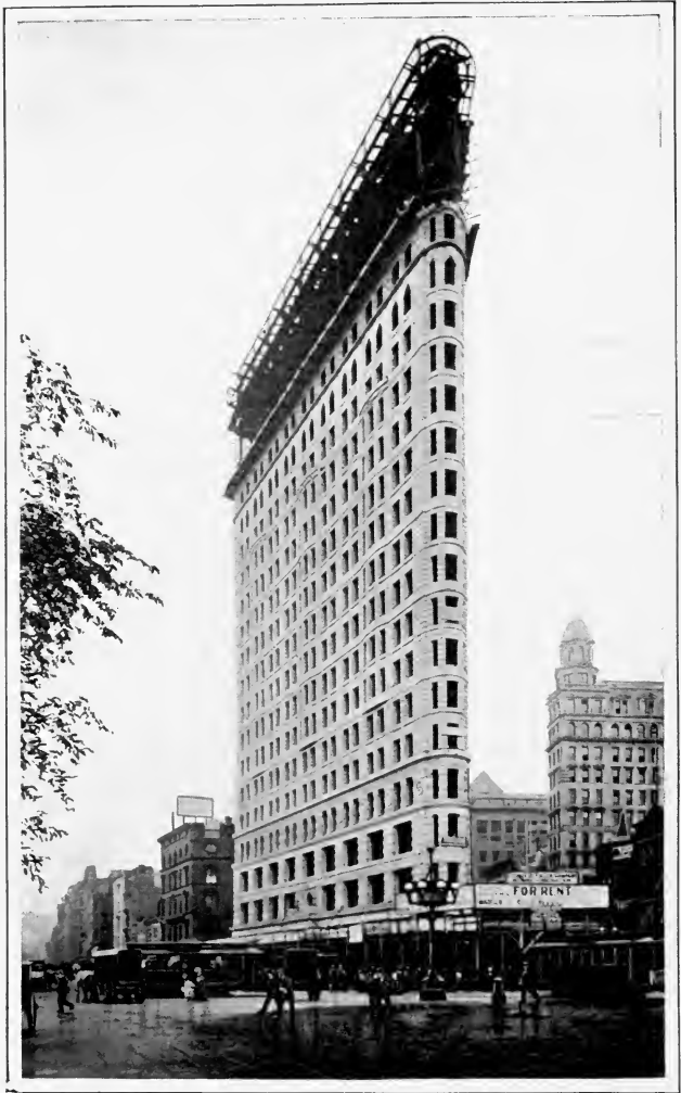
THE "FLAT-IRON" NEARING COMPLETION
