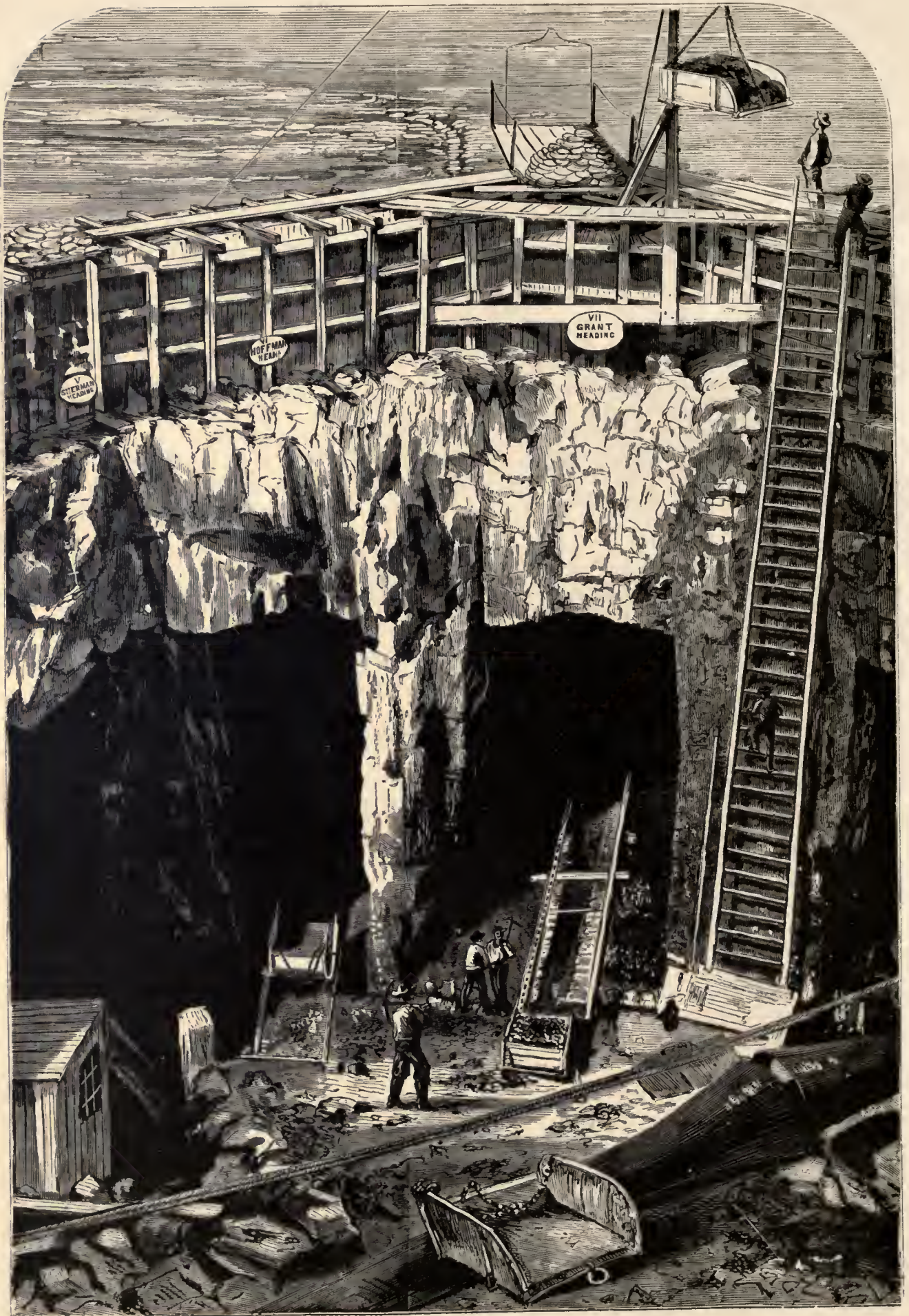
OPENING OF THE SHAFT BENEATH HELL GATE.
