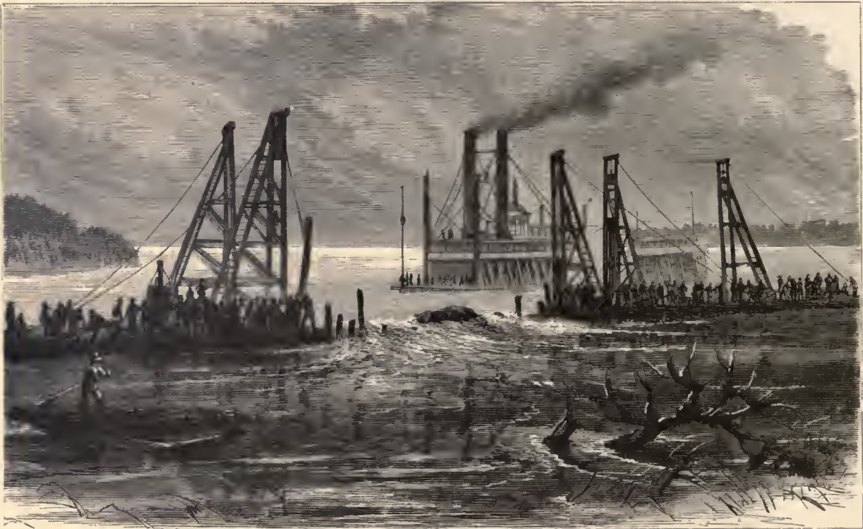
Removing Snags by Dredging.
