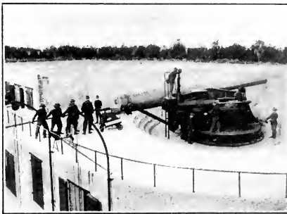
LOADING A DISAPPEARING GUN, WHEN IT IS IN THE DEPRESSED POSITION.
