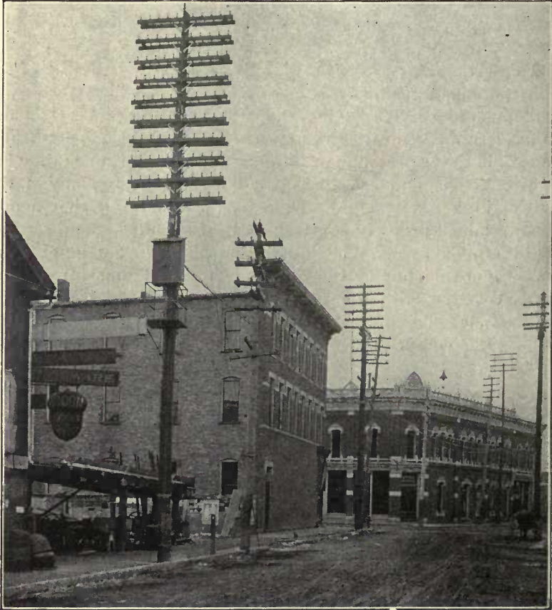
Fig. 326.—Cable Terminal Box with Balcony.
