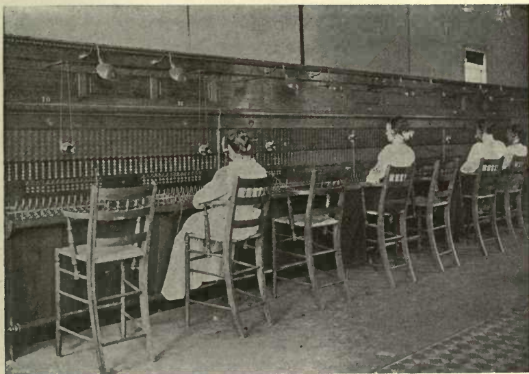
Fig. 192.—800-Line Sterling Switch-Board.
