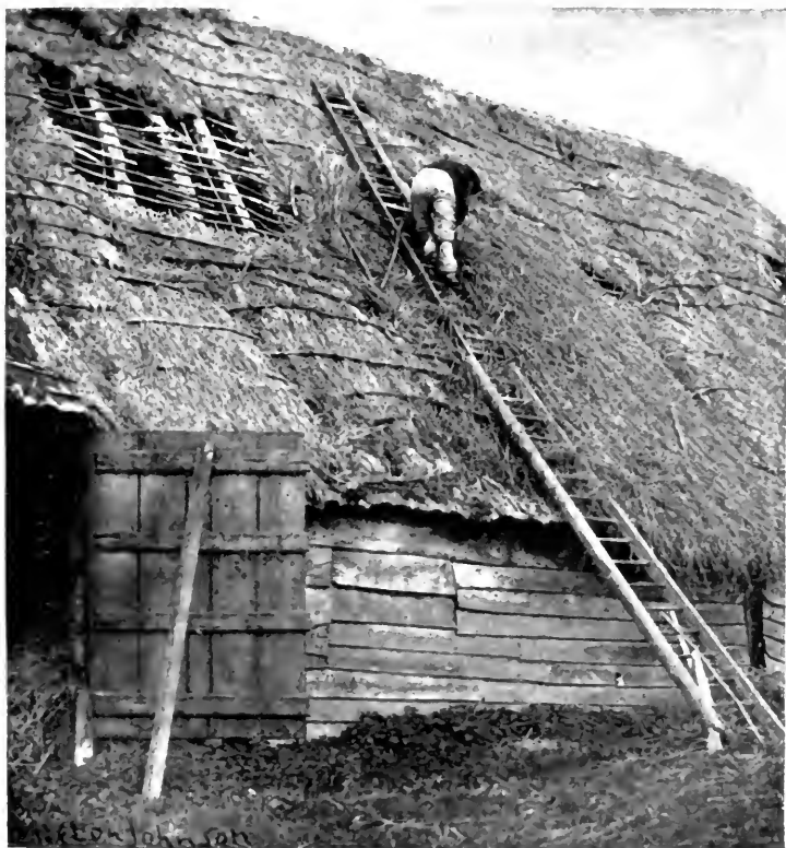
Patching the Thatch Roof of a Barn
