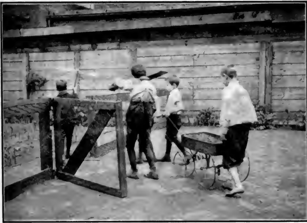
HAULING STREET SWEEPINGS, LOUISVILLE, KY.
