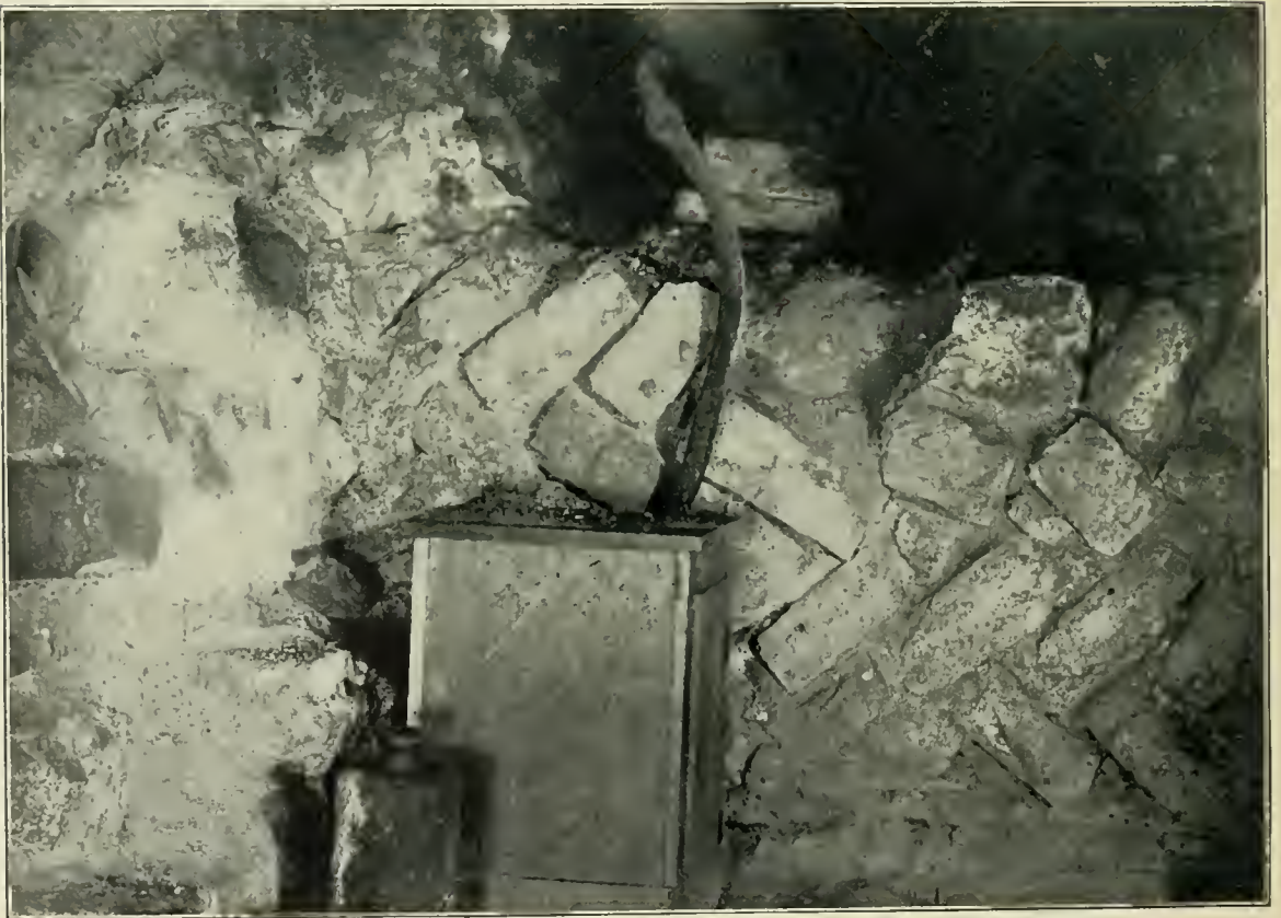
THE SOUTH WALL.
