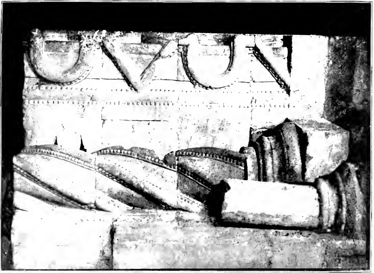
PORTION OF A DOOR
