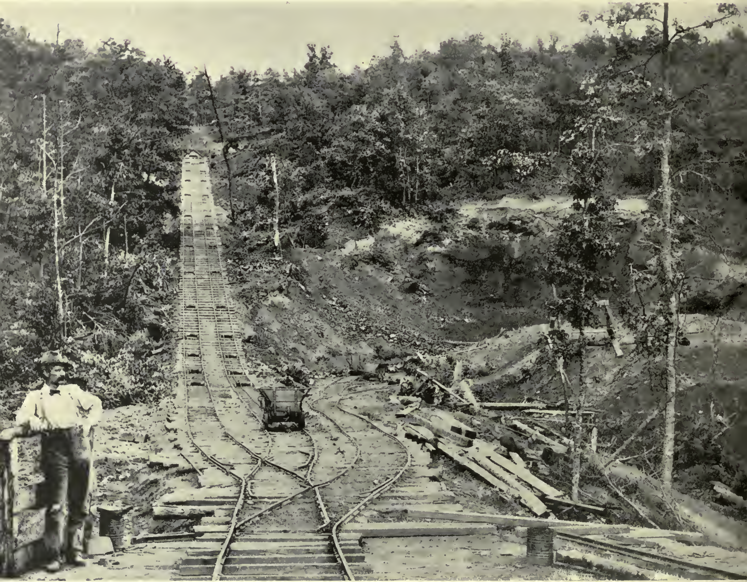
HUDDLESTON MINE, POTTS VALLEY, VA., SHOWING INCLINE.
