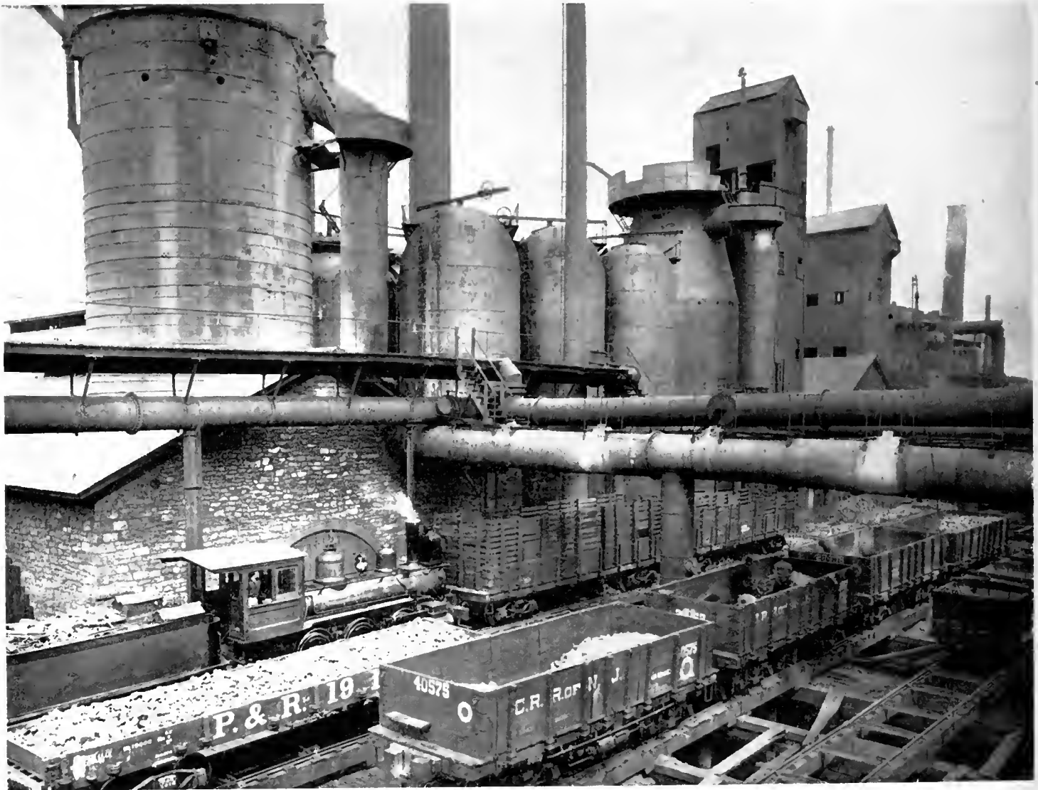
CRANE IRON WORKS, SHOWING UNLOADING OF ORE.
