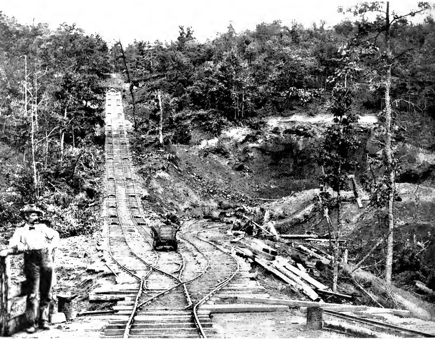
HUDDLESTON MINE, POTTS VALLEY, VA., SHOWING INCLINE.
