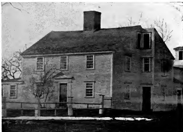
ISAAC DAVIS'S HOUSE NORTHBORO, MASS., 1775 to 1850.
