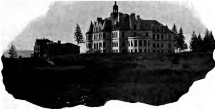
ADMINISTRATION BUILDING UNIVERSITY OF WASHINGTON SEATTLE
