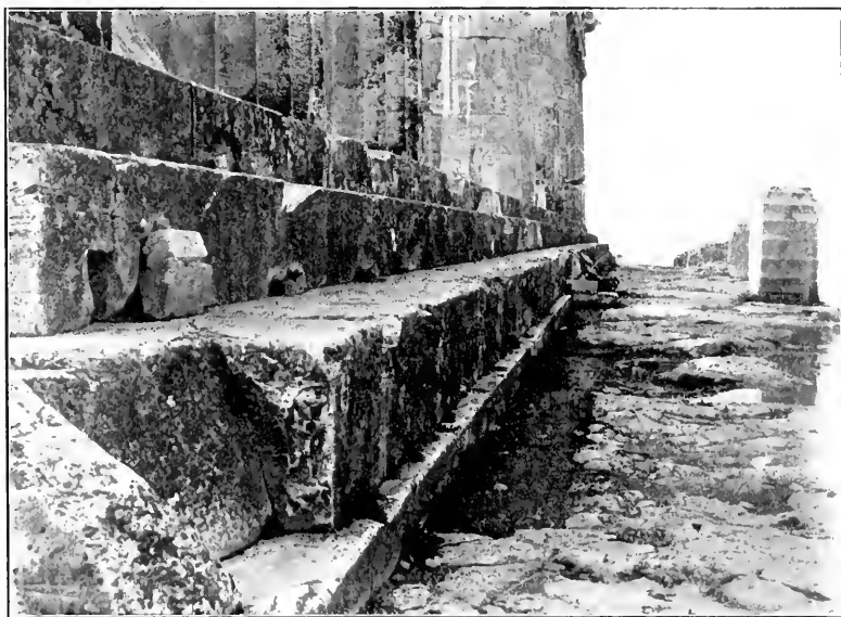
NORTH SIDE OF PARTHENON, SHOWING CURVE OF STEPS.
