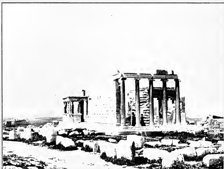
ERECHTHEUM FROM THE SOUTH-EAST.
