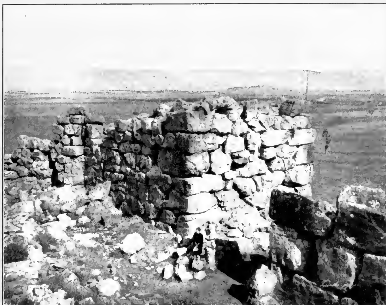
WALL AND TOWER AT TIRYNS.
