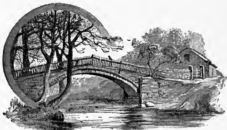
BECKFOOT BRIDGE, BINGLEY.
