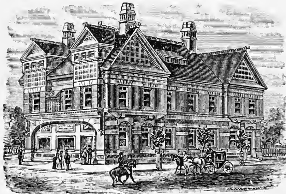
MUTUAL FIRE INSURANCE BUILDING, GERMANTOWN.
