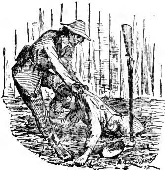
IGNOMINIOUS END OF A TUNNEL ENTERPRISE.
