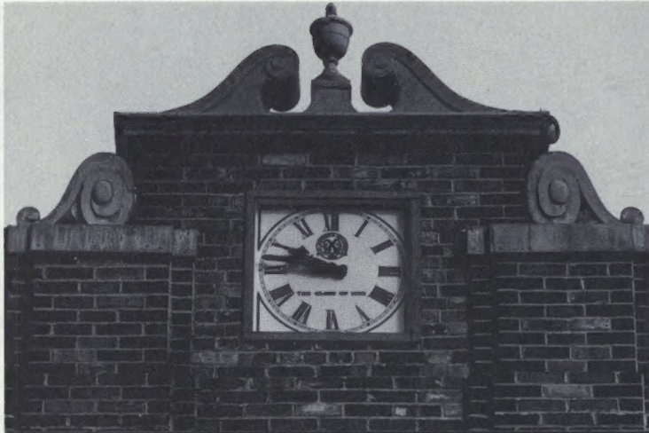
The Class of 1993 donated a new clock for Dunlap Hall as their leaving gift to S.A.C. Installed in the fall of 1993, the clock is a very elegant addition to the administration building.
