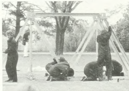
Demonstrating the portability and erection of a 24' wooden bridge capable of carrying 1400 lbs. is a group of Grade 13 cadets who designed and constructed the bridge themselves.
