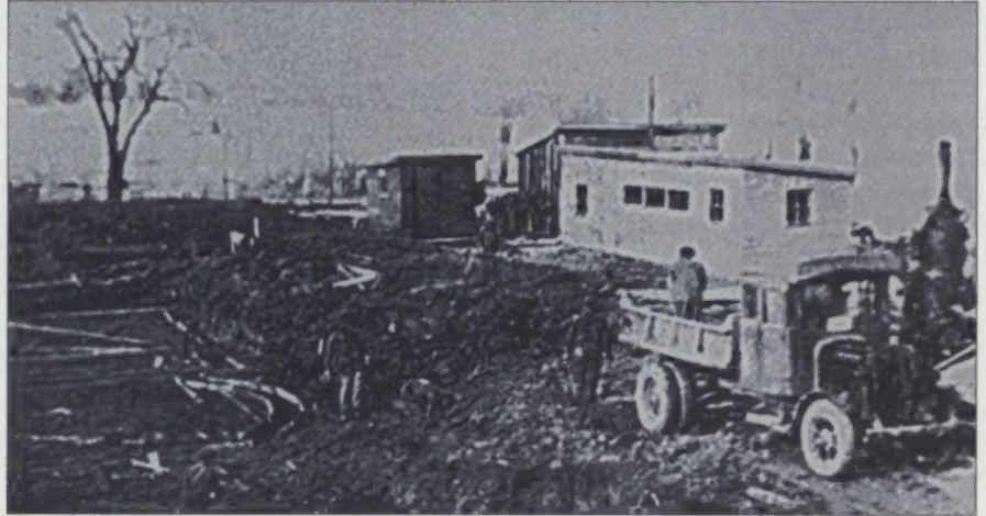
Foundation work on new Lower School Building
