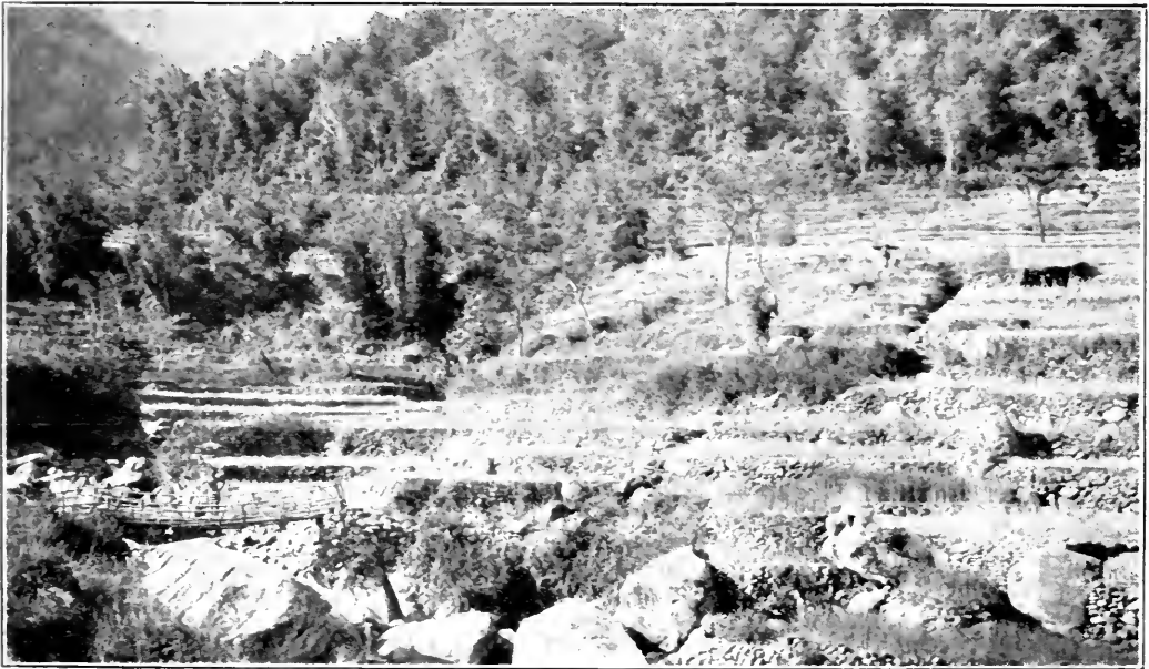
TERRACING AND BRIDGE AT KHONOMA
