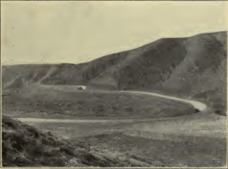
PLATE II.—Main south canal, Uncompáhgre Valley. Lined canal section through clay foothills.
