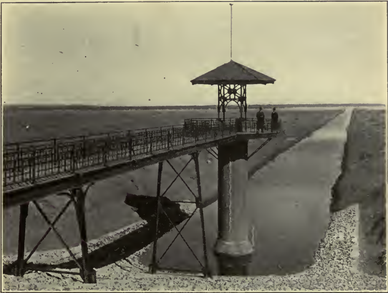
PLATE VI.—Outlet tower, Hondo reservoir, New Mexico.
