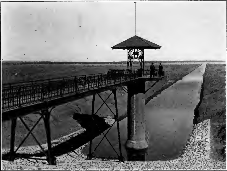
PLATE VI.—Outlet tower, Hondo reservoir, New Mexico.
