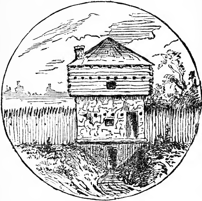
Block House. Built in 1780.
