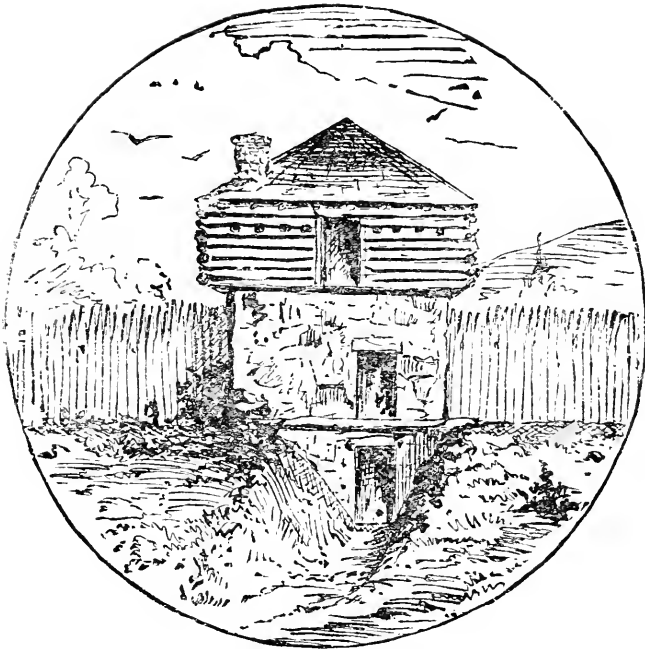
Block House, Built in 1780.
