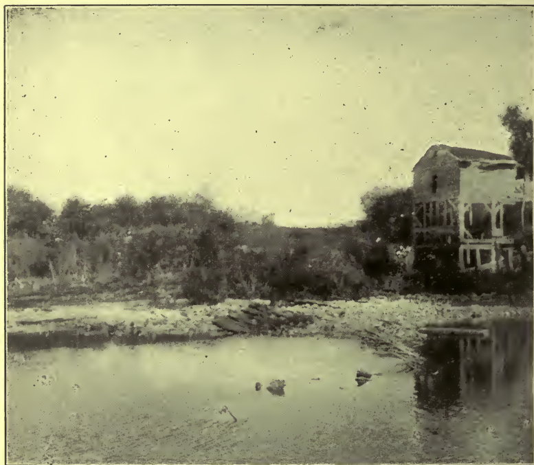
THE HEDDLESTON-SIGLER-COLTRAIN MILL, CEDAR TOWNSHIP.
