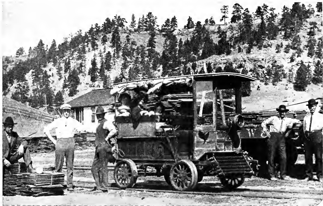
One of the road's two "dinkys" pulls out of Aladdin with a full load aboard.
