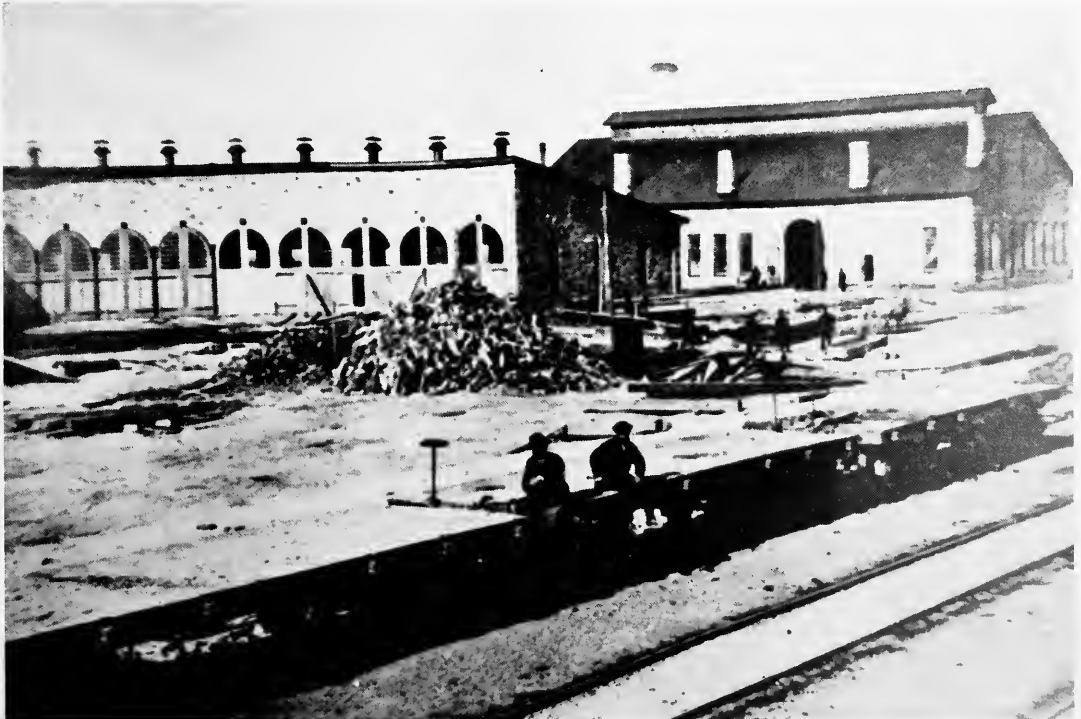
Newly constructed railroad shops at Laramie, circa 1870.
