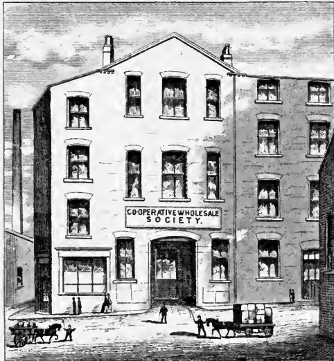
LEEDS SALE AND SAMPLE ROOMS, 58, ALBION STREET.
