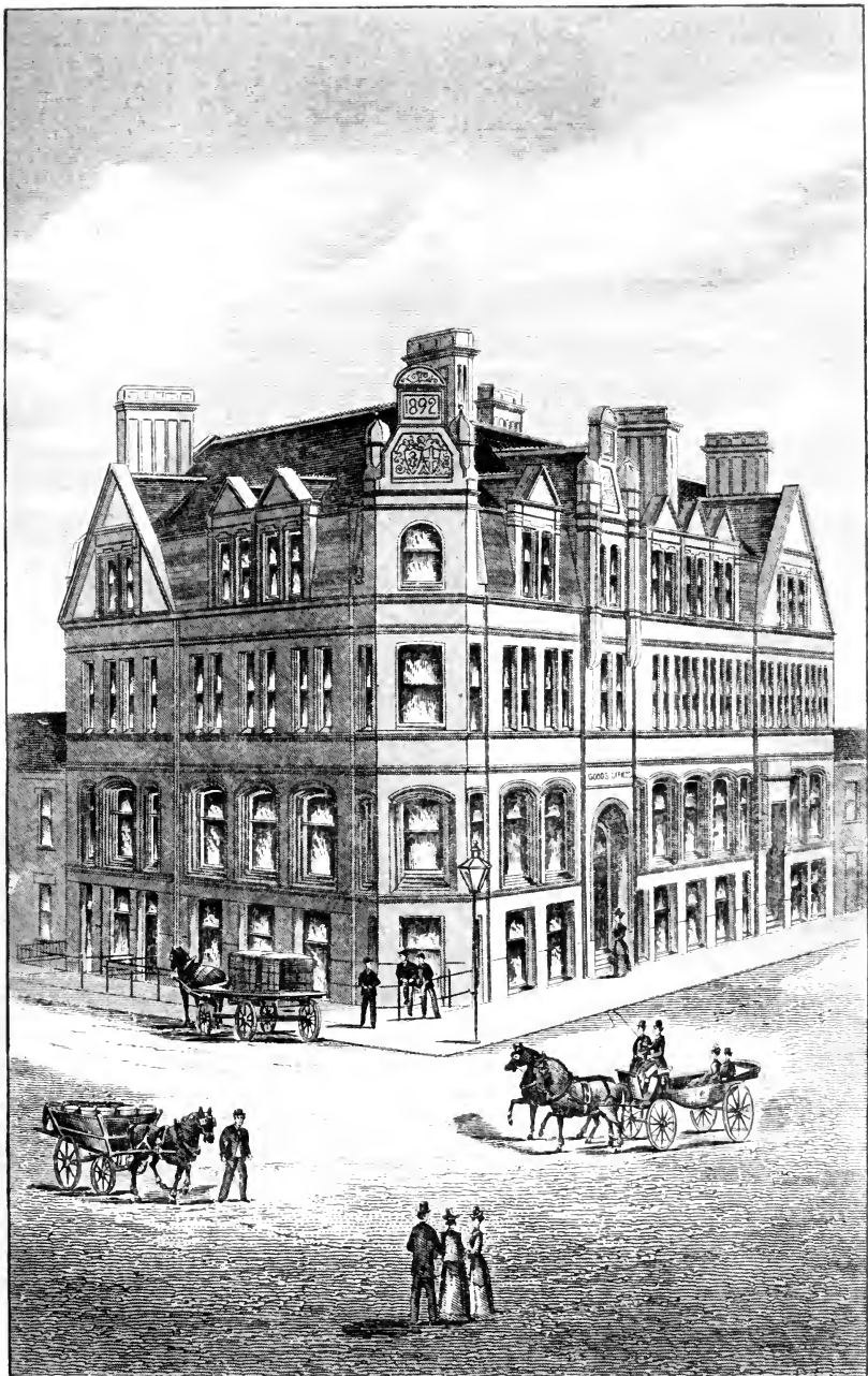
GOOLE OFFICES, STANHOPE STREET.
