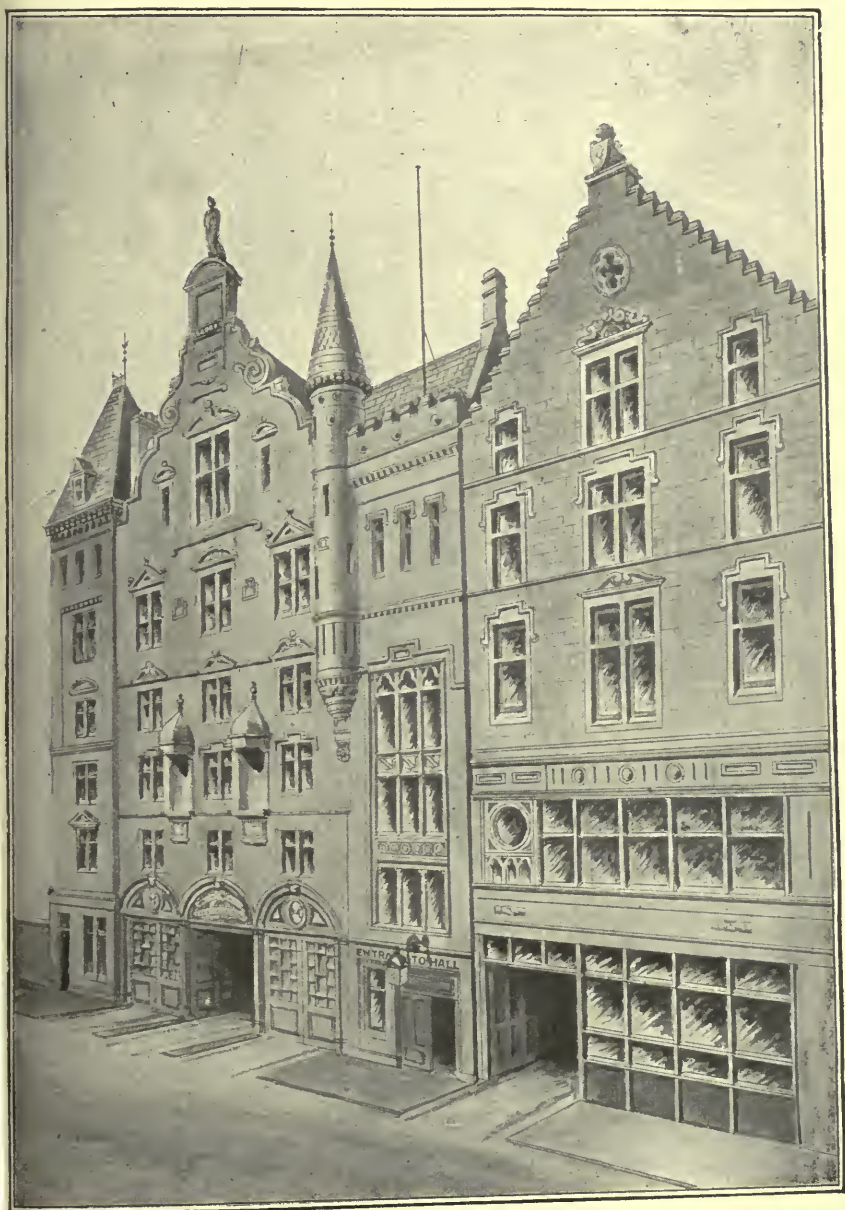
GROCERY AND PROVISION WAREHOUSE AND HALL, CLARENCE STREET, GLASGOW
