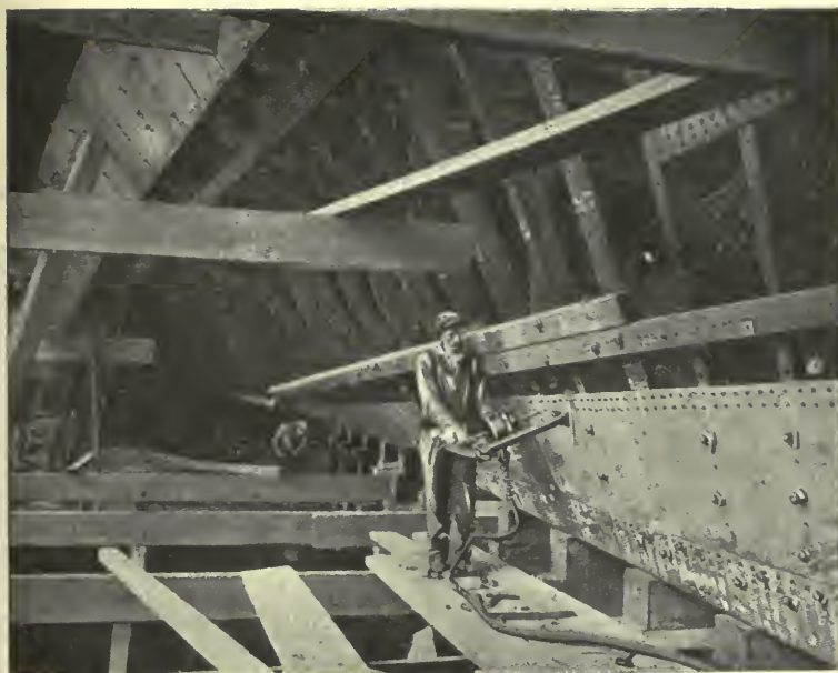
DRILLING ON SHIP HULL WITH PNEUMATIC DRILL.
