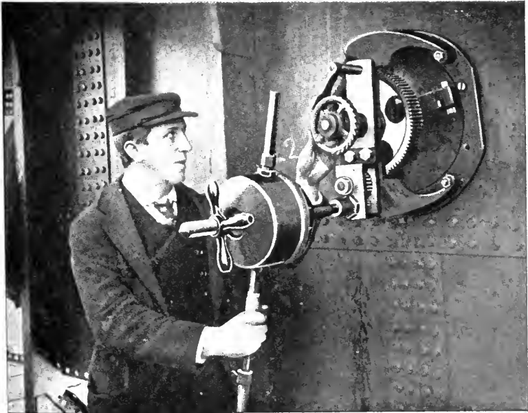
SIDE-LIGHT CUTTER IN CONNECTION WITH DRILL.
