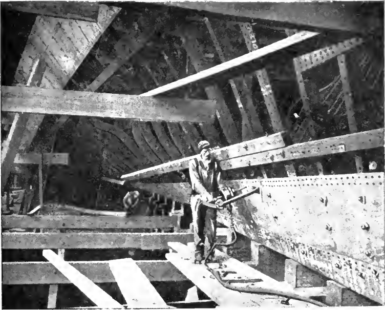
DRILLING ON SHIP HULL WITH PNEUMATIC DRILL.
